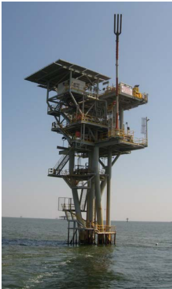
Gulf of Mexico Oil & Gas Platform
